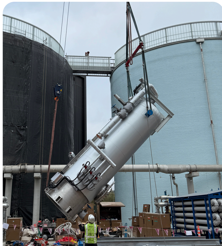
THP pressure vessel being installed at the Southeast Treatment Plant in San Francisco, CA (USA)
